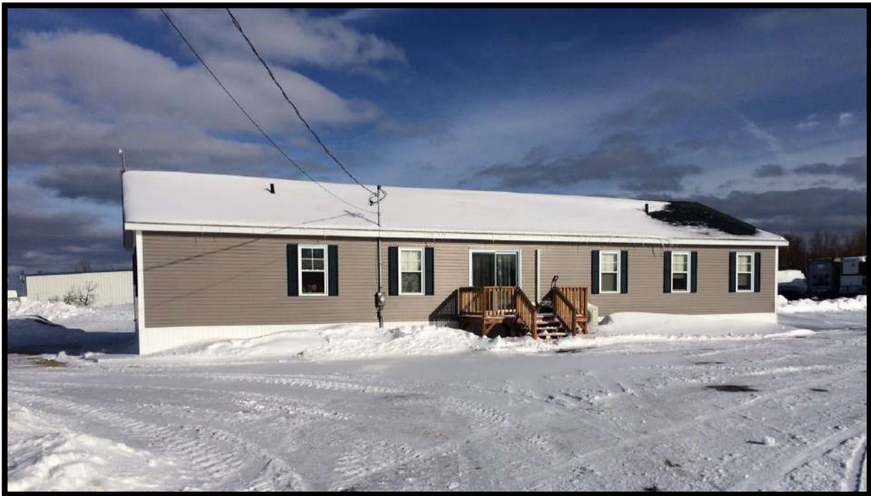
Figure 10: New Lodging Building, Local Service District of Escuminac
