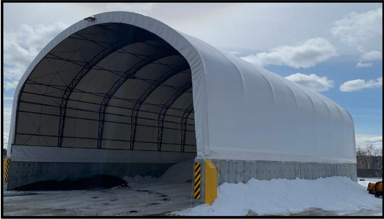
Figure 5: New Salt Storage Dome, Village of Doaktown
