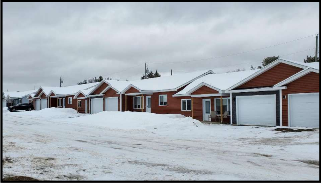
Figure 7: New Rowhouses, City of Miramichi
