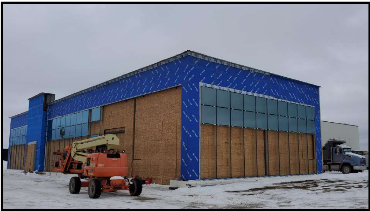
Figure 6: Commercial Building Construction, City of Miramichi
