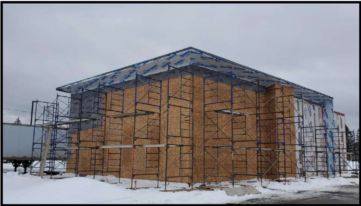
Figure 8: Restaurant Construction, City of Miramichi
