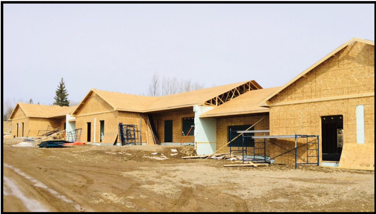
Figure 7: Rowhouse Construction, City of Miramichi
