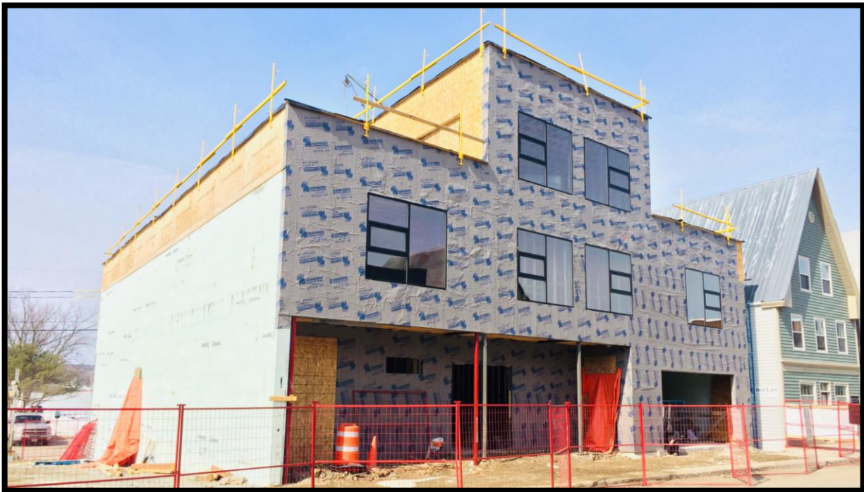
Figure 9: Office Building Construction, City of Miramichi
