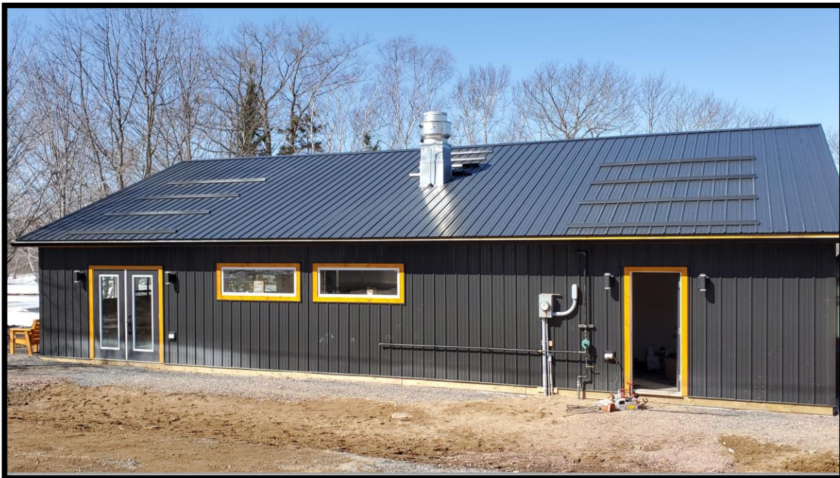
Figure 5: Restaurant Construction, Village of Doaktown
