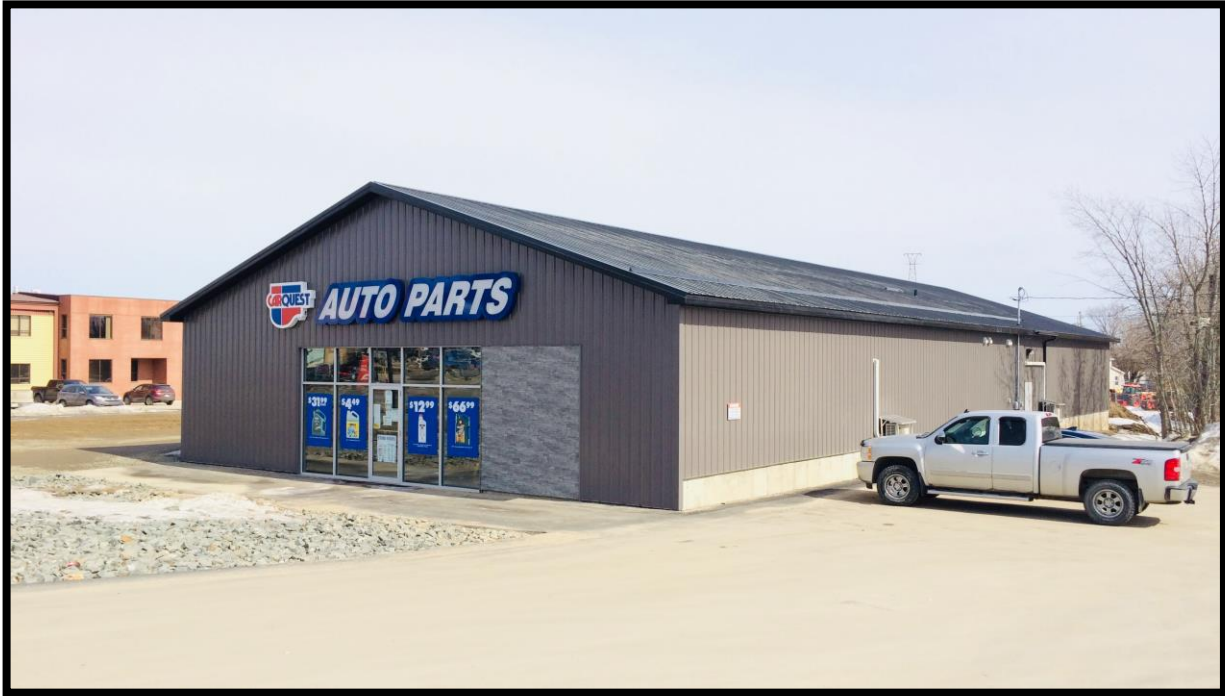
Figure 6: New Commercial Building, City of Miramichi
