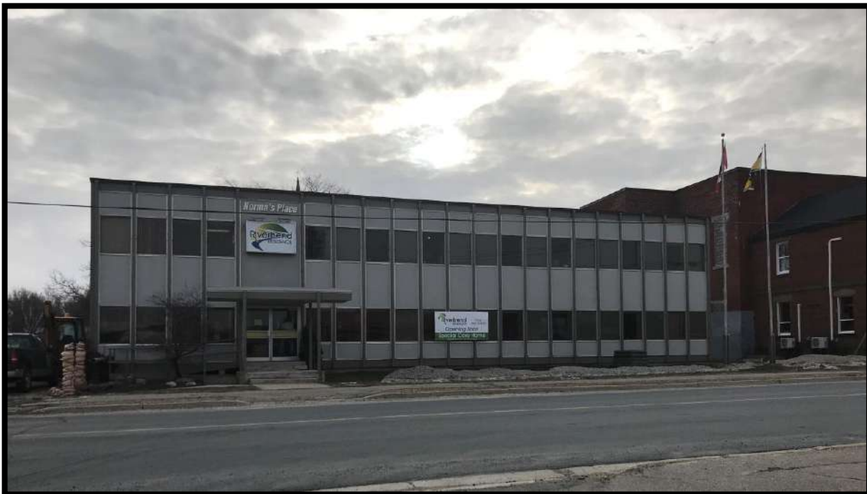
Figure 6: Office Building Conversion to a Special Care Home, City of Miramichi
