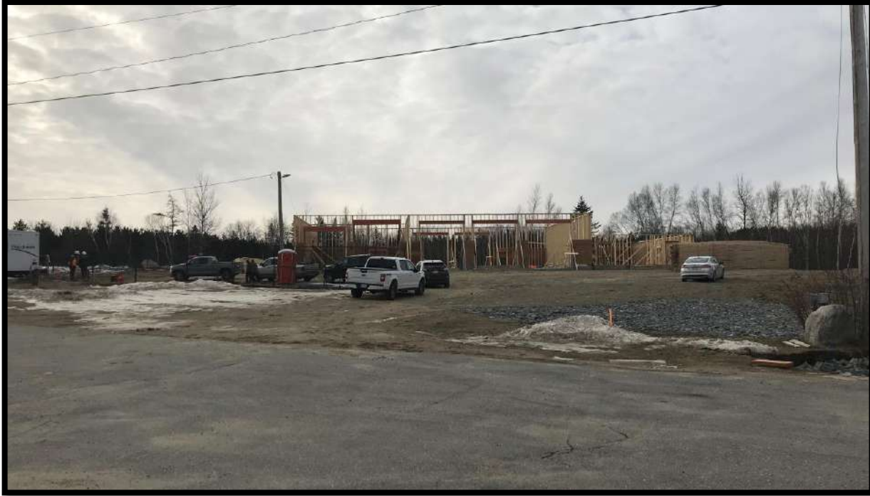
Figure 5: Fire Hall Construction, L.S.D. of Renous-Quarryville
