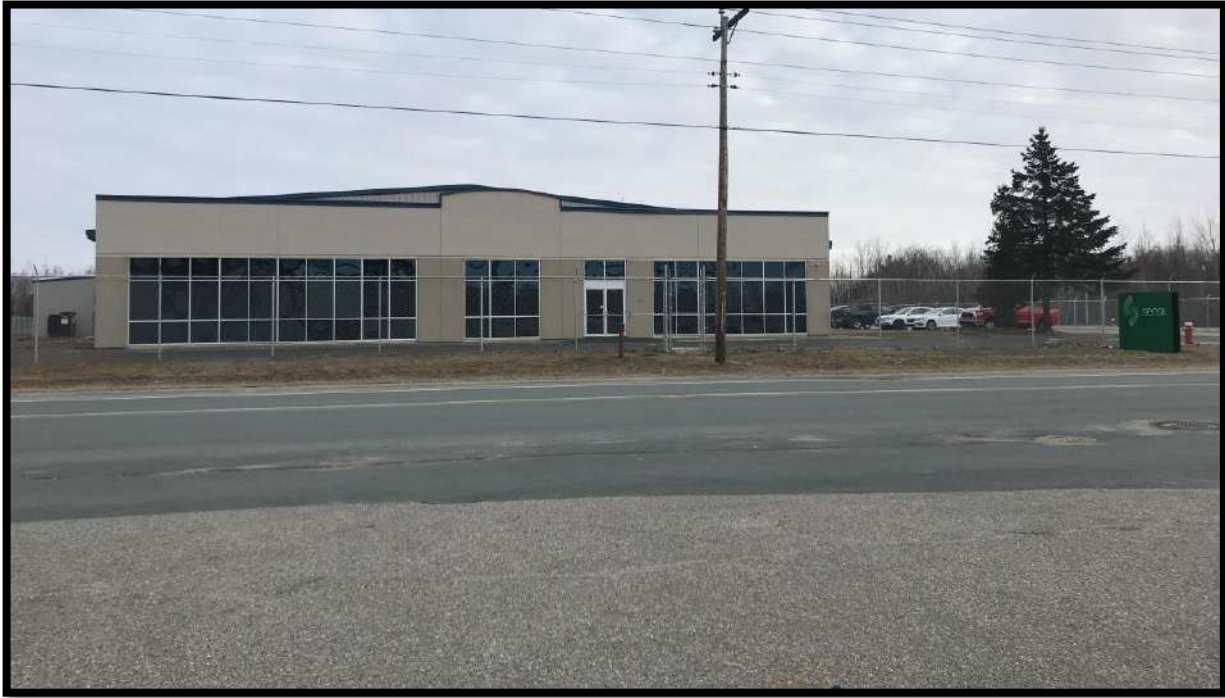
Figure 9: Cannabis Production Facility, City of Miramichi
