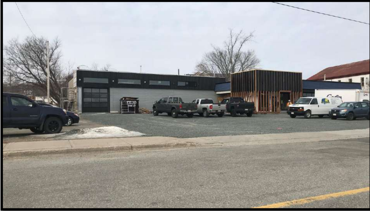
Figure 7: Glass Repair Shop Conversion to a Brewery, City of Miramichi
