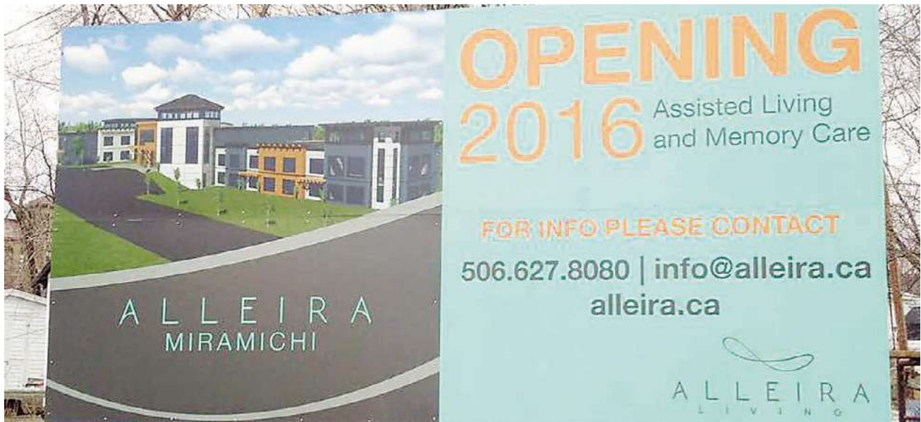
This billboard positioned on the former St. Mary's convent property shows designs of an incoming 96-bed specialized-care facility that will feature a number of beds reserved for people suffering from dementia. PHOTO: ALLEIRA LIVING
