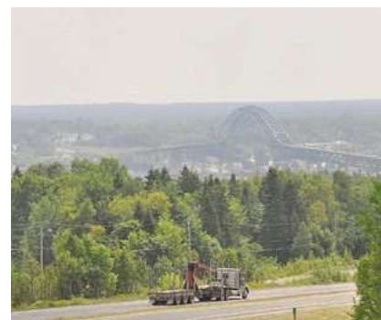
The Centennial Bridge.
