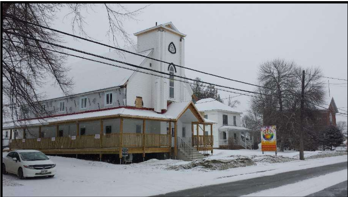
FIGURE 11: FORMER ST. MARK'S CHURCH TO INSTRUCTIONAL CLAY WORKING CAFÉ, CITY OF MIRAMICHI
