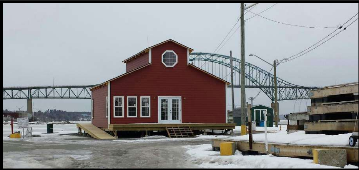
FIGURE 14: STATION WHARF MARINA OFFICE BUILDING, CITY OF MIRAMICHI
