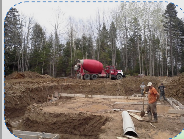
E.g. Foundation excavation
