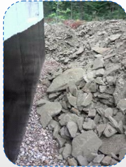
E.g. Drain tile and granular fill
