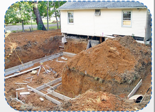
E.g. Foundation excavation
